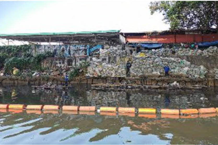
Along Sevilla Bridge (boundary of Sta. Mesa, Manila and Mandaluyong City)
