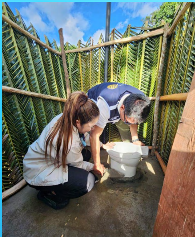
DG Joyce Ambray and yours truly installing a toilet bowl.
