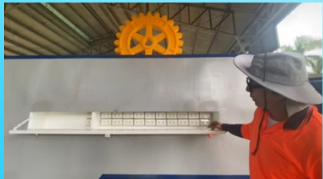
On the left side is the phone and laptop charging station to keep the community connected even when power is out
