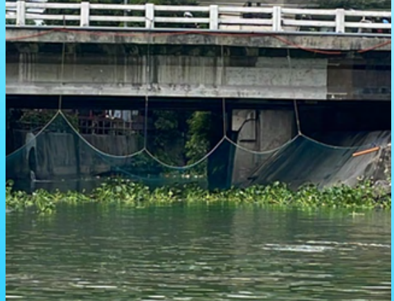
Waste traps installed were not enough to prevent all the trash from going into the river.
