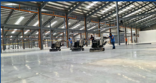
Concrete Polishing System
