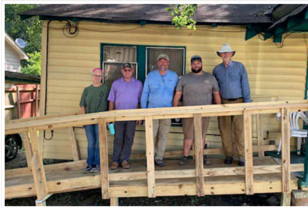
— Members of the Rotary Club of Henderson, Texas, spend their Saturday building a wheelchair ramp.
