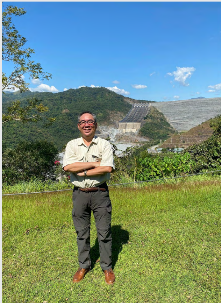
At San Roque Hydro Power Station, another Marubeni project in the Philippines
