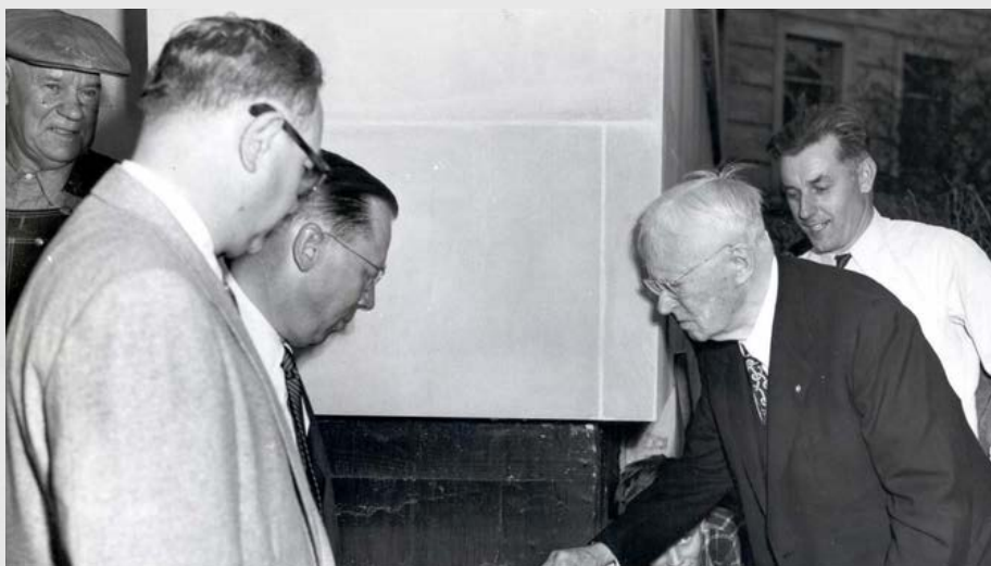
Guy Gundaker (with trowel), 1923–24 RI president, prepares to lay the cornerstone of the Ridge Avenue building in Evanston, Illinois, USA. 1954.
