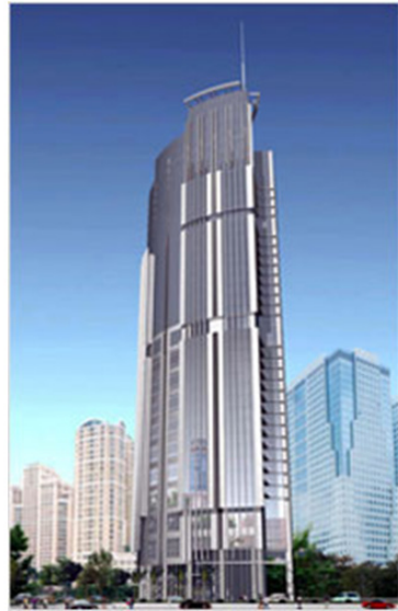
Figure 3 54 Storey One Corporate Center, Ortigas Ctr
