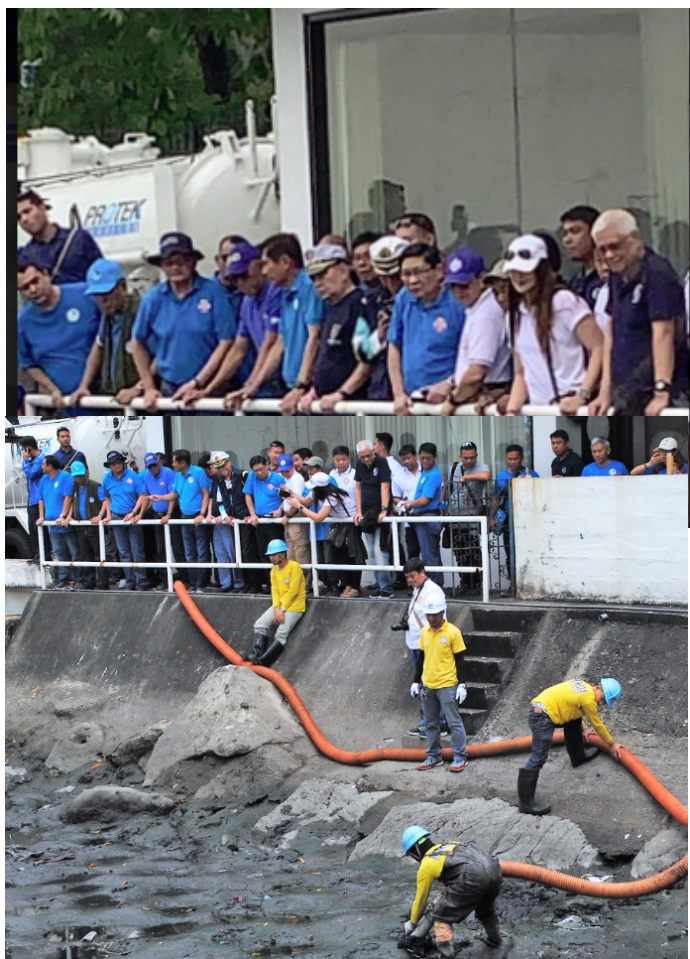
The dredging at the Manila Yacht Club
