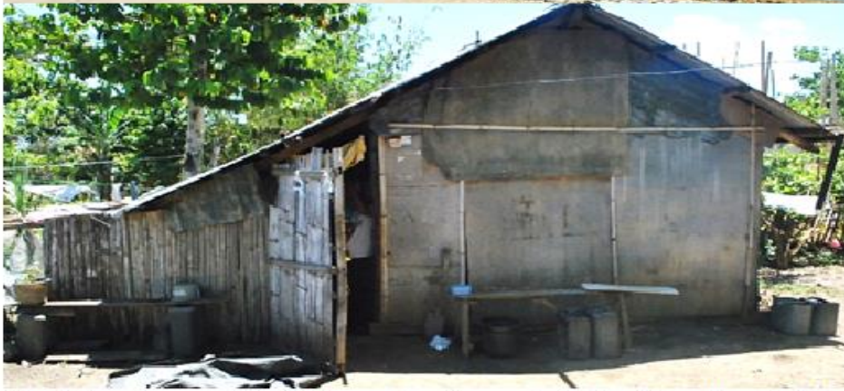
The 30 row houses (at right) construction cost of Php 4.5 million, built by Gawad Kalinga and funded by Governor KAI (Rotary Japan) , Rotary Clubs of Bangkok, Osaka-East, Kowloon-East and RC Manila . Bottom photo shows former house structure of the beneficiaries.
